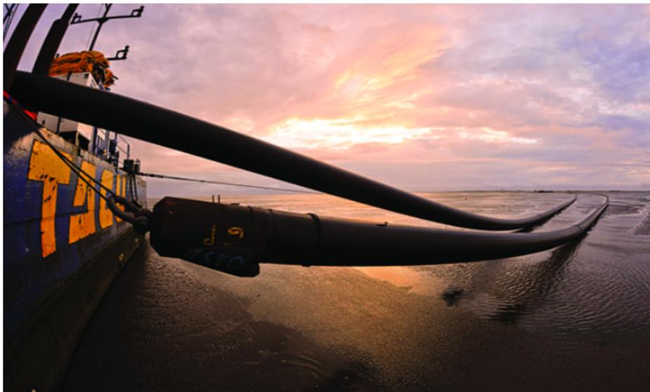
FIGURE 1.5: Power generated by the Nordsee One, Gode Wind I, and Gode Wind II offshore wind farms is transmitted to land via HVDC subsea cables [10].
