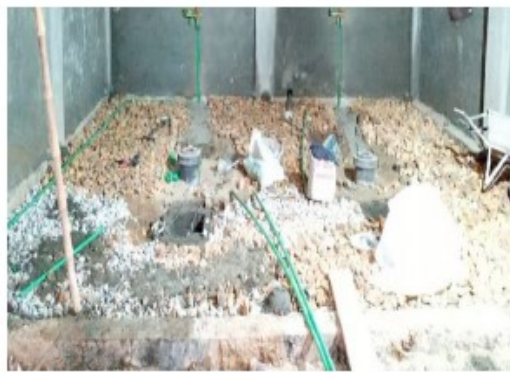
c. Reuse of Brick Blast in Flooring
