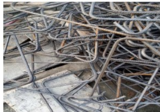
e. Use of Steel Pieces for Hooks and Stirrups
