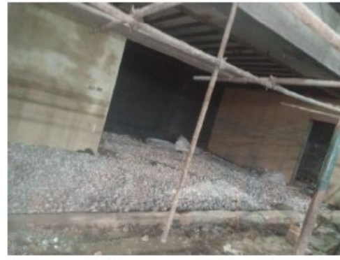
d. Reuse of Concrete as Filling Material
