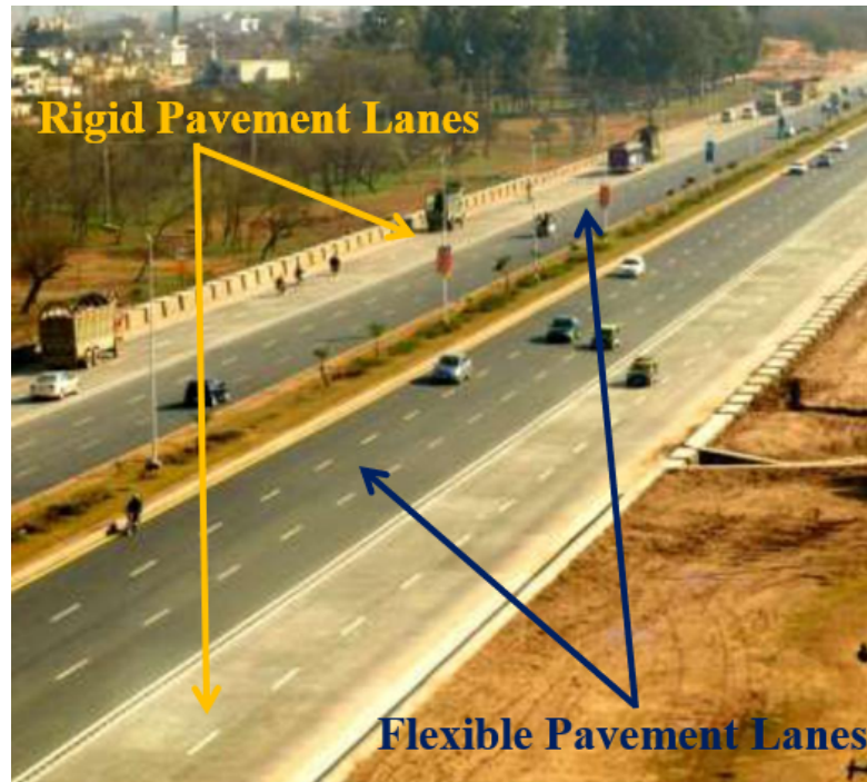
FIGURE 2.1: Existing flexible and rigid pavement lanes in road network of Islamabad, Pakistan.
