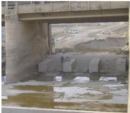
FIGURE 3.6: Existing appurtenances of barrage [43]
