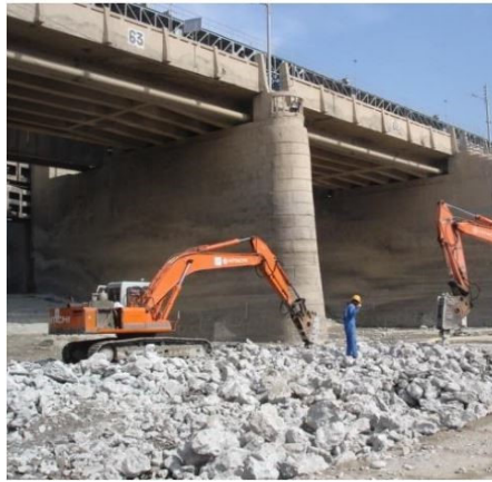
FIGURE 3.5: Dismantling of Baffle blocks [43]
